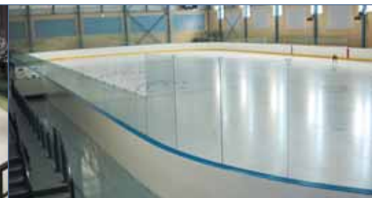
National Ice Centre, Nottingham. 60m x 30m Community & Arena Pads.
