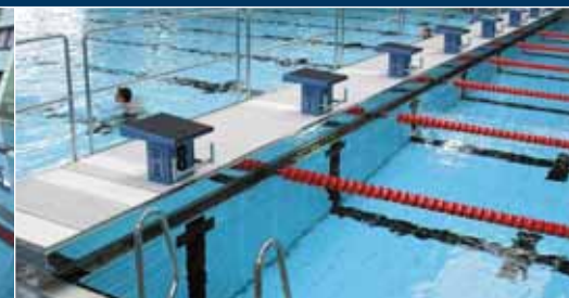
Loughborough University. The traversable boom design allows for speedy movement.
