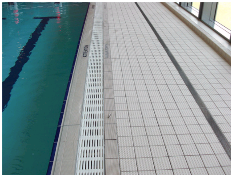
BS EN 15288 compliant pool surround with central ACO channel at Cambletown pool, Scotland
